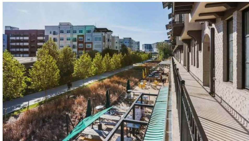
Figure 13: The Residences at Studioplex, situated above ground-floor BeltLine retail.
