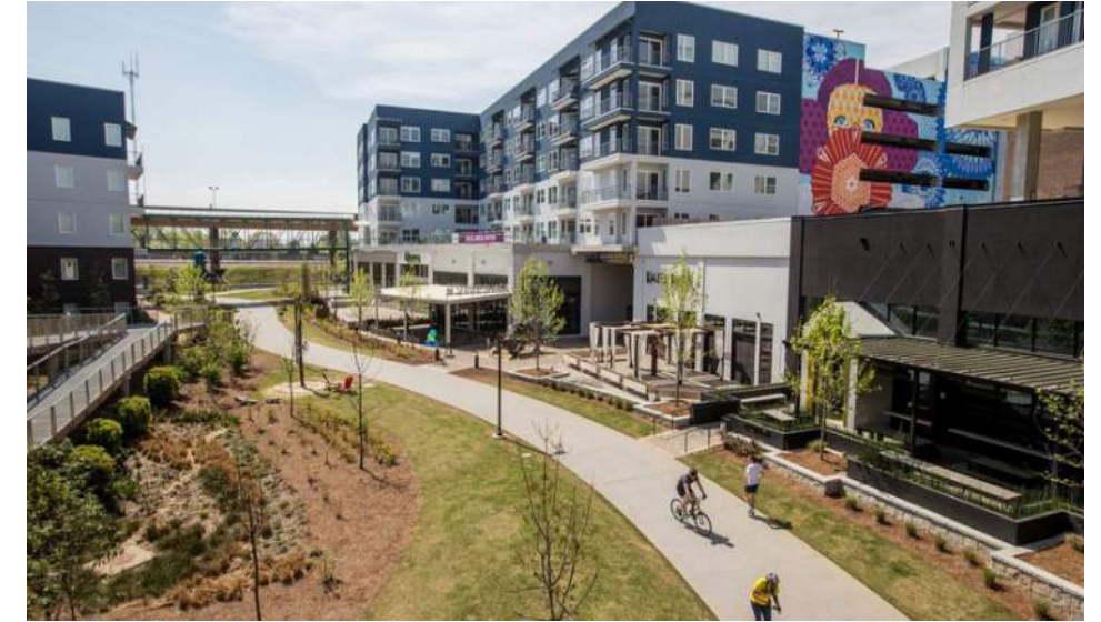
Figure 14: A multifamily development on the southern edge of the Eastside Trail.
